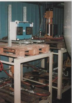
Fully automatic SNR plant for ammonia solution, delivered at Ena Kraft, Enköping, Sweden.
